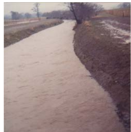
Stokesley diversion channel in action, shortly after it was built in the 1970s
